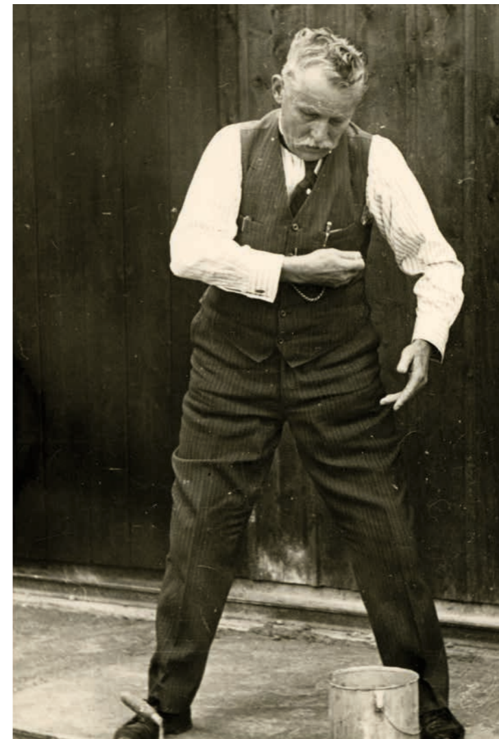
Kaspar Winkler preparing a mix of Sika®-1 for demonstration purposes
