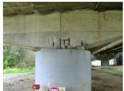
Atmospheric carbonation induced corrosion
