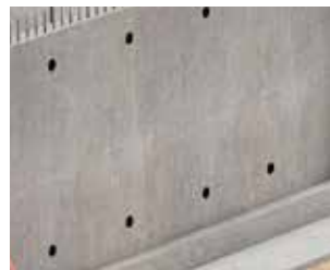
SikaSwell® Rings and Plugs Sikadur® 31 Sealing tie bar holes
