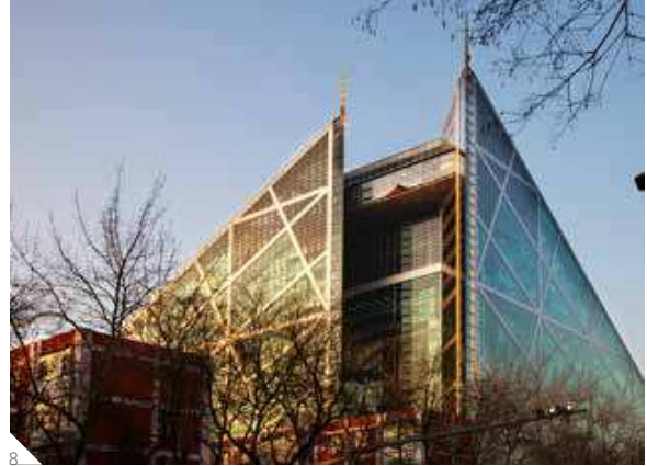
65 Park View Green Plaza, Beijing (2010) Consultant: ARUP Hong Kong Facade by Beijing Jianli (CN)
