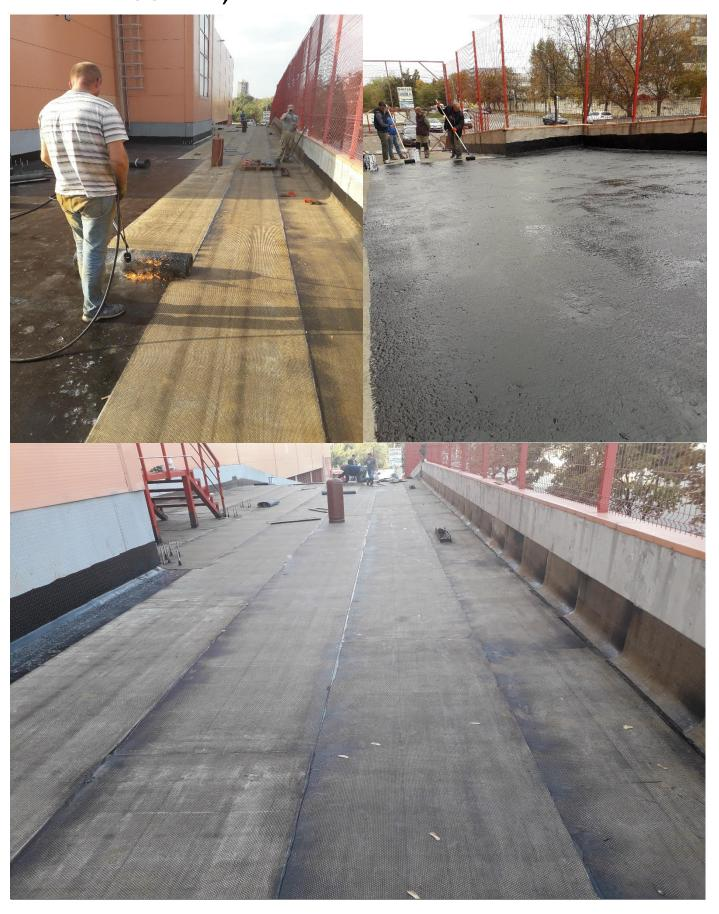
**PROJECT DESCRIPTION:** On the facility has successfully completed the waterproofing of the loading ramp of one of the Auchan stores. Was used bitumen primer Sika Igolflex P-10 and the polymer bitumen membrane Sikabit P50-15 HR30. The system used provides for further laying on the membrane of hot asphalt. The project was implemented together with the partners company – Penetron MK. Waterproofing area is 1800m2.
