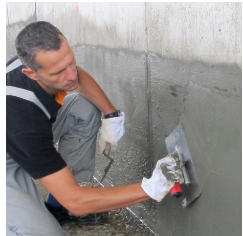
PCI Barraseal has a creamy consistency, pores and cavities can be closed easily and rapidly.
