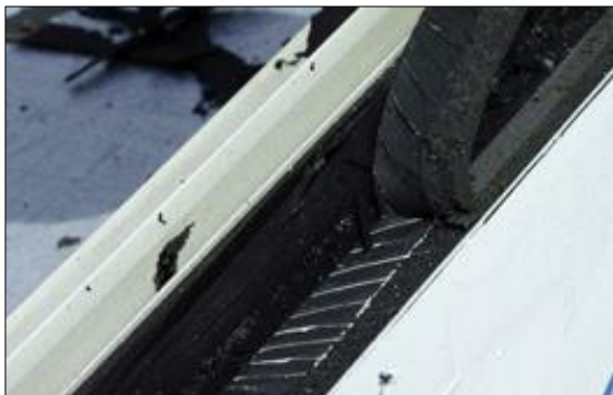
Figure 39: Example with black SG joint - Good adhesion.
